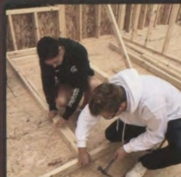
Sydney Hintz and Oliver McCarthy building a wall for the house Oliver and Ryan Bickle designed.
