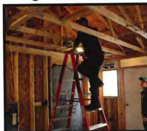
Working on trusses.
