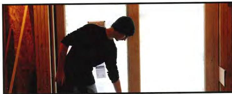
Finishing the sliding doors.
