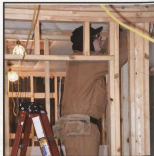
Working on trusses.
