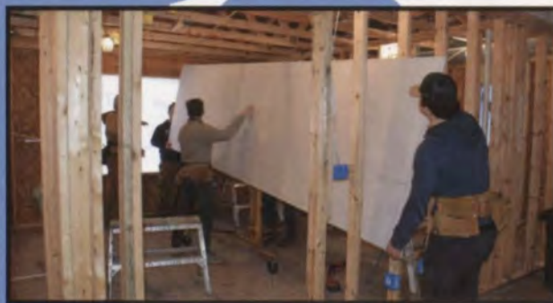
Applying drywall.
